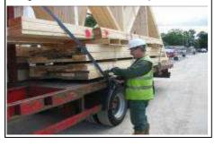
5. The operator must position the forklift in an appropriate area to ensure the trusses are lifted safely. The forklift will take the weight of the trusses on the forks ensuring no one is within the danger area.
