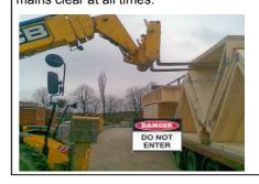
7. The driver will cut the individual rope / banding attaching the pack to the bars. This must be carried out from a safe position using a telescopic cutting staff.
