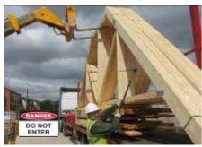
8. The forklift truck operator must lift the trusses from the trailer and then move the trusses to a safe and / or off-load area.
