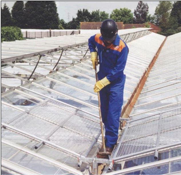
Figure 13 Valley walker used during gutter cleaning. This provides a protective mesh covering to either side of the operative, which moves progressively along the roof as the worker moves forward. The protective covering eliminates the risk of a fall through the fragile material (Image courtesy of Safesite Limited)
