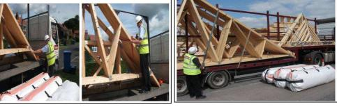
8. The driver will apply a wedge between the 1st and 2nd truss. The driver will then re-fit one of the small straps through the gap to secure the pack but leaving one to be taken by the customer.
