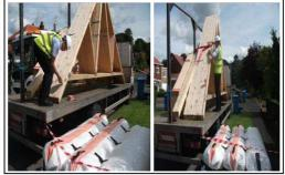
9. The customer shall place his team to receive the truss. The customer shall remove the truss from the vehicle. The driver will repeat this method by releasing one truss only.
