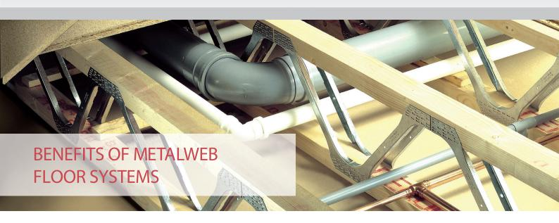
Constructed of kiln dried stress graded timber and plated together with high strength steel webs, metalweb floor systems have a number of benefits compared with other floor and joist systems.
