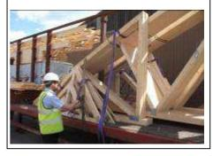
7. The driver will cut the individual rope / banding attaching the pack to the bars. This must be carried out from a safe position using a telescopic cutting staff.
