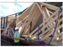
8. The crane will then lift the truss pack from the bed of the trailer. **NEVER** stand in the danger area where the trusses could potentially fall. Do not allow any others to enter the danger area.
